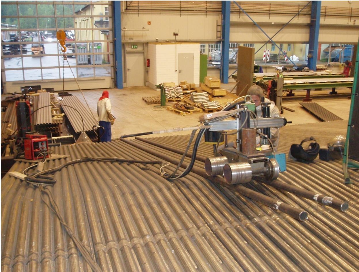
Post cladding of shop assembly seams
