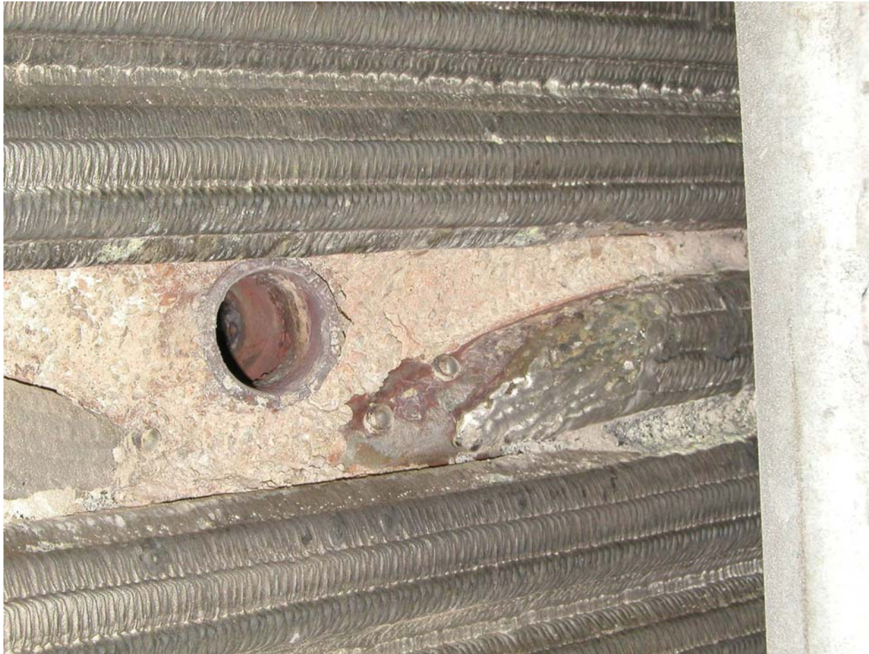
Chipped refractory in area of bendings
