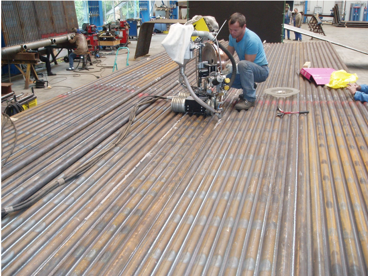
Assembly of cladded panels in the width
