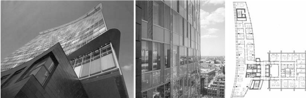
Figure 2 The Gemeinnützige Siedlungs- und Wohnungsbaugesellschaft (GSW) Headquarters, (1999) in Berlin, Germany was designed by Sauerbruch Hutton Architects and Arup (HVAC/energy consultant). The 22 story tall building is characterised by a double facade towards the west that utilises solar energy to boost the thermal buoyancy in the cavity, which in turn suck air out of the building. Fresh air is provided through a myriad of ventilation inlets in the east facade. The plan of the highrise is narrow (11.5-15 m) to facilitate utilisation of daylight and natural ventilation 4, 5, 6 .
