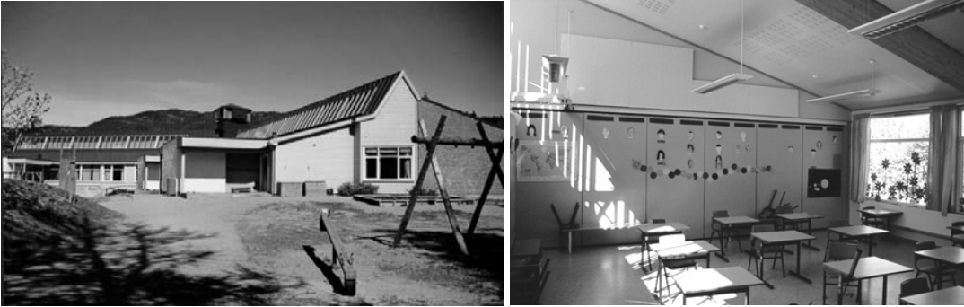
Figure 4 The Mediå Primary School, (1998) in Grong, Norway was designed by Letnes Architects AS and VVS Planconsult AS (HVAC/energy consultants). The school is characterised with an exhaust chimney and a combined sunspace/extract chamber on the roof. The sunspace provides the classrooms with extra daylight, increases the thermal buoyancy and enhances the efficiency of the recovered heat from the exhaust air. An embedded duct connected with an inlet tower provides fresh air into the interiors 10, 11 .
