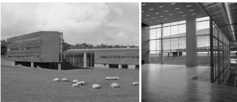
Figure 3 The Bang & Olufsen (B&O) Headquarters, (1998) in Struer, Denmark was designed by KHR AS Architects and Birch & Krogboe AS (HVAC/energy consultant). The naturally ventilated southern office wing is characterised by being elevated as well as having an extremely light appearance from the court (made possible by the absence of suspended ceilings and ducts familiar to mechanical ventilation systems). The north facade of this wing also has a band of narrow openable windows in front of each floor slab serving as ventilation inlets. The interior spaces are used as airpath. Two stairwells are used as extract chimneys. The ventilation concept is totally integrated in the building structure, the building appears not to have a ventilation system at all 7, 8, 9 .
