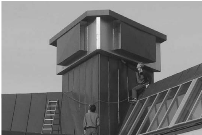
Figure 9 Installation of measurement tube on the roof tower wall.
