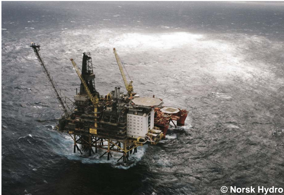
Gas and Oil extraction from the offshore platform “Oseberg C”
