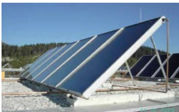
FIGUR 4-2 Takmontert solfangerpanel.
