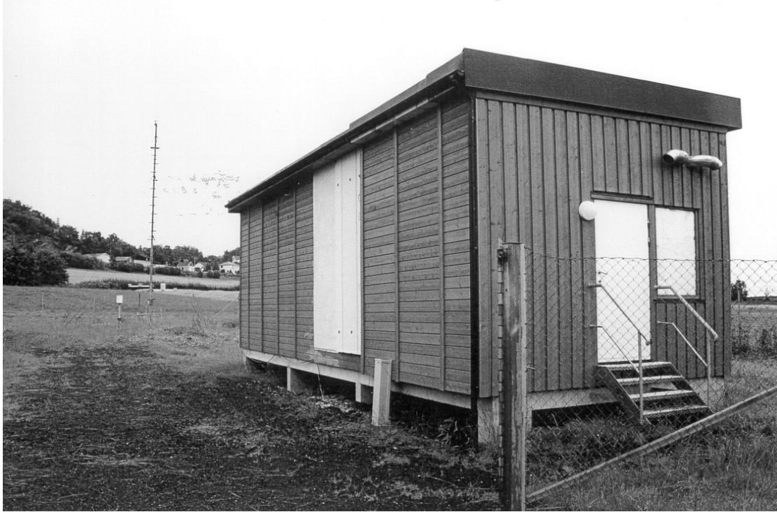
Figure 2 The northeast side of the test house.
