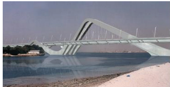
Figure 4-2: Sheik Zayed Bridge, Abu Dhabi. Lower part of supports are of reinforced concrete with steel type 1.4462 in the outer layer of reinforcement /32/
