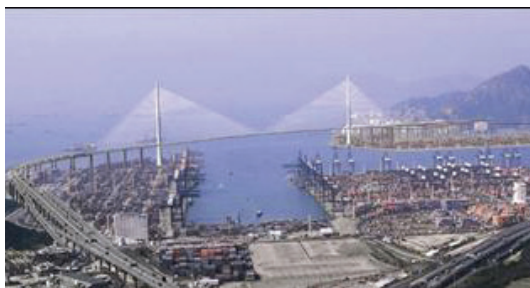
Figure 4-1: Stonecutters Bridge, Hong Kong. Pylons reinforced with steel type 1.4462 in the outer layer of the multi-layer of reinforcement /32/
