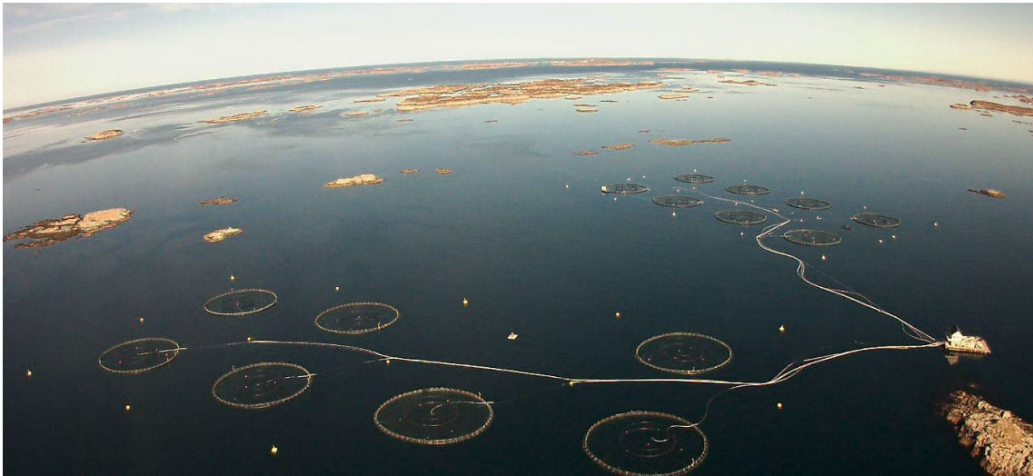
One of the full-scale test sites at SINTEF ACE
