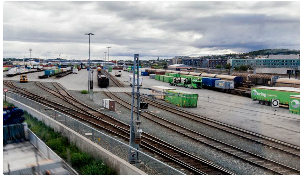
Glimpse of the transport system: Trondheim freight terminal.
