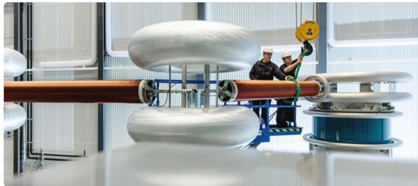
High up: Installation of experiments in the high-voltage hall at SINTEF Energy Lab.
