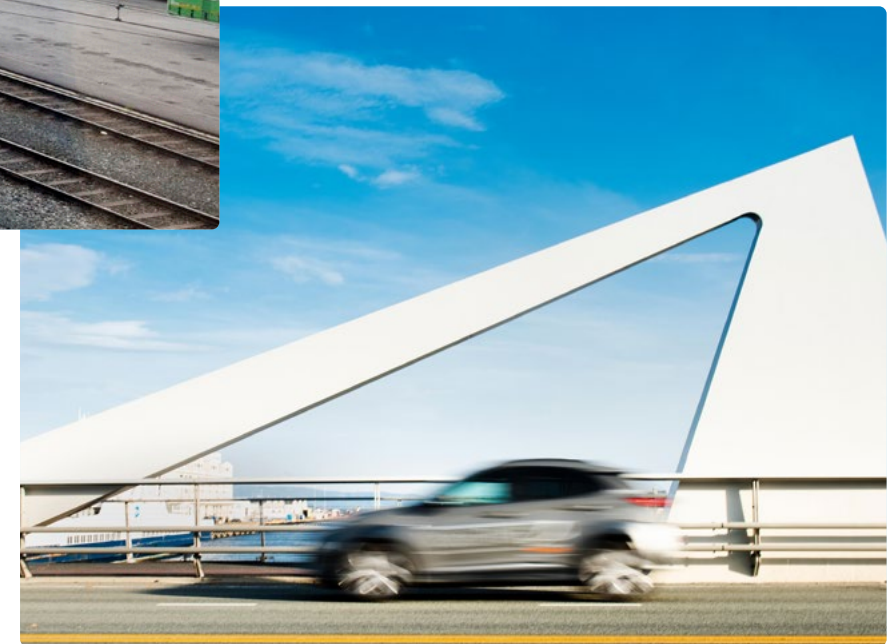
Glimpse from the road network: Pirbrua in Trondheim.
