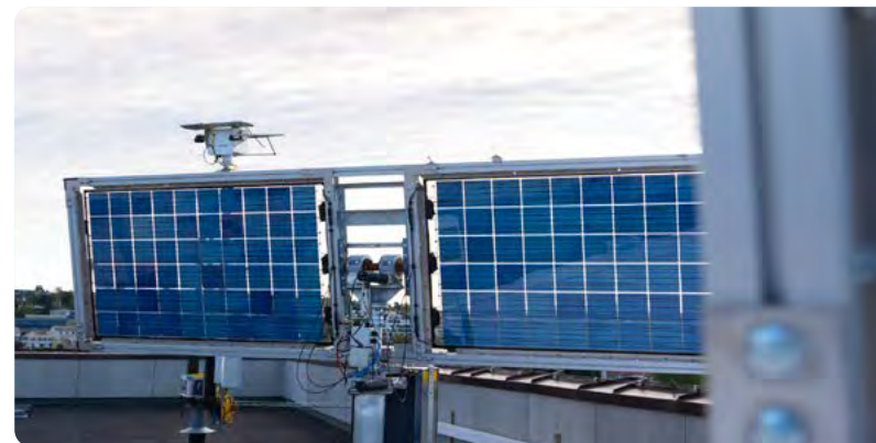
Double-sided solar panels that trap sunlight directly and from the surrounding environment. The solar panels follow the sun's location in the sky with the help of a solar tracker.
