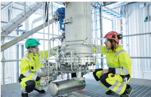
Gasification reactor in the combustion laboratory at SINTEF Energy Lab.
