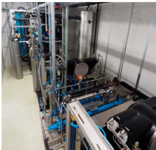
Interior of the 10 t/d CO 2 liquefaction and separation pilot facility
