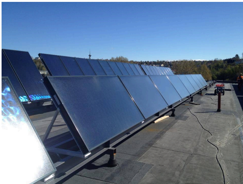
Figure 14 Solar thermal array at Scandic Hotel Lerkendal.
