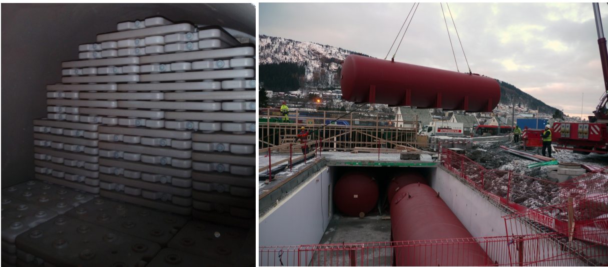
Figure 16 PCM elements inside the cold storage tanks (left) and cold storage tanks being placed underground at the Bergen University College (right) [27].
