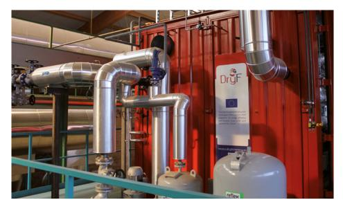
*Figure 9:* Heat pump developed within the framework of the DryFiciency project (AT)
