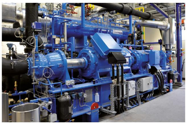
Figure 7: Heat pump installed at the Marienhütte steel and rolling mill Source: 17
