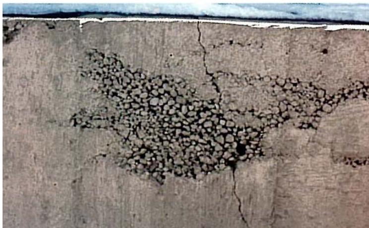
**Figure 5:** Example of honeycombing (PCA IS536.01 2002)
