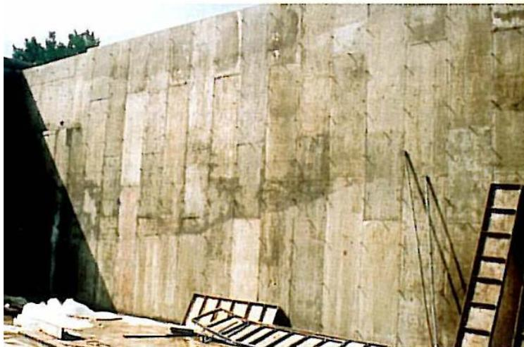
**Figure 4:** Cold joint illustrated by a sloping horizontal line (PCA IS536.01 2002)
