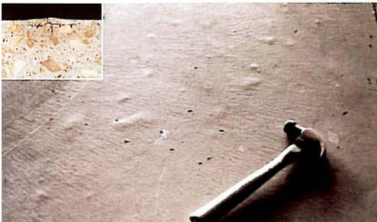
**Figure 7:** Delaminations and blisters (PCA IS536.01 2002)
