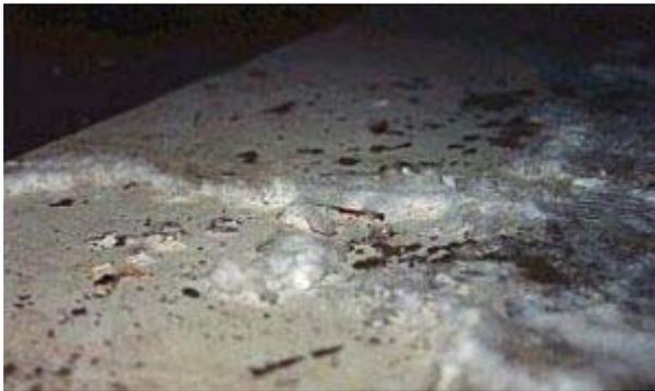
**Figure 1:** Efflorescence
