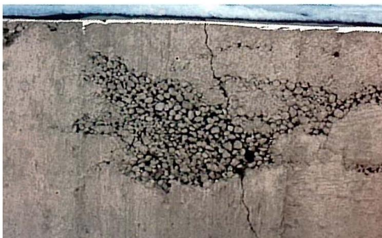
**Figure 5:** Example of honeycombing (PCA IS536.01 2002)
