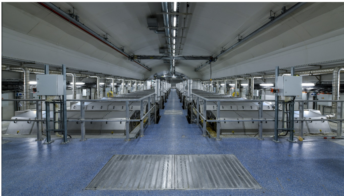
Figure 4: HydroTech drum filters at IVAR SNJ (Photo: Kjetil Birkedal Pedersen, IVAR)
