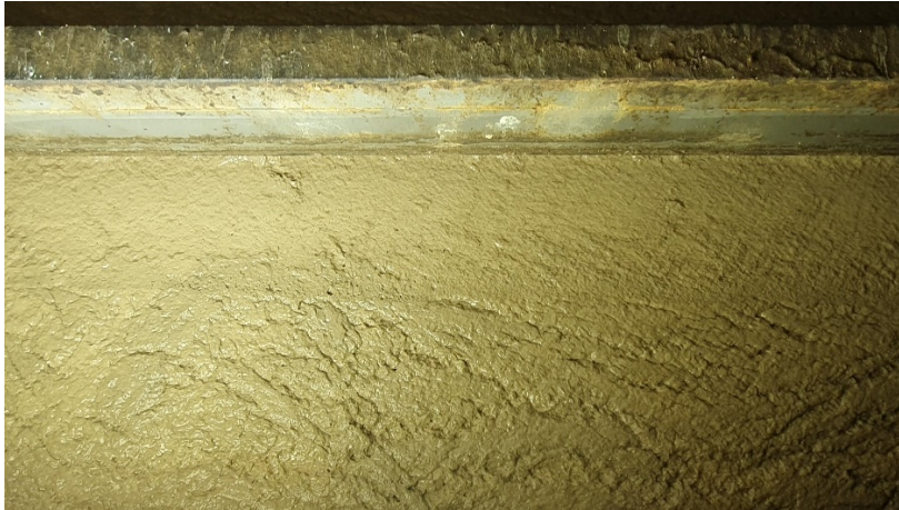
Figure 2: Sludge blanket with the sludge scrape
