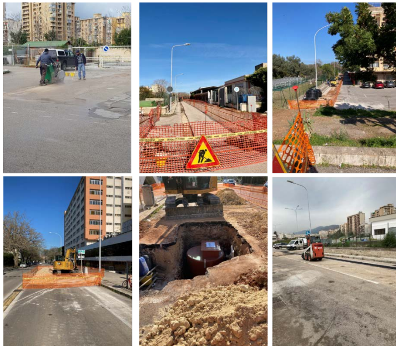
Figure 22: HDPE pipeline and fiberglass polyester tank during installation
