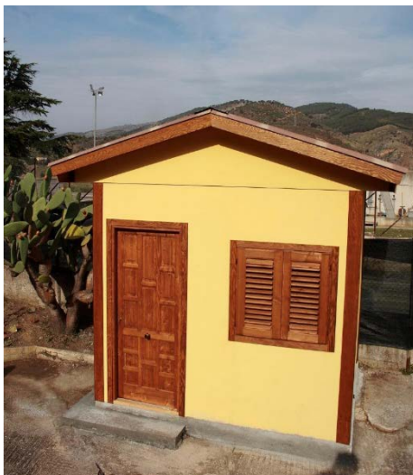
Figure 2 New shed for PHA extraction line at Marineo's Wastewater Treatment plant.
