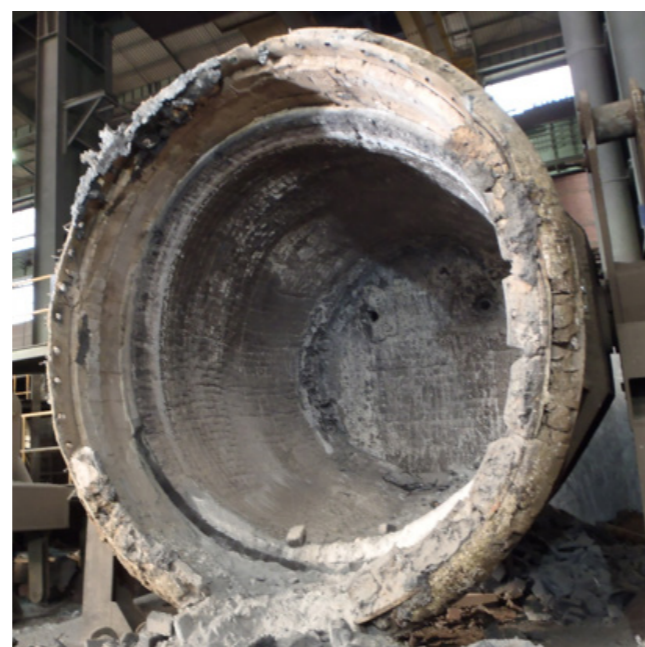
Ladle with slag lining demolished
