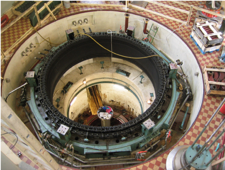
Fig. 6. Generating unit pit.
