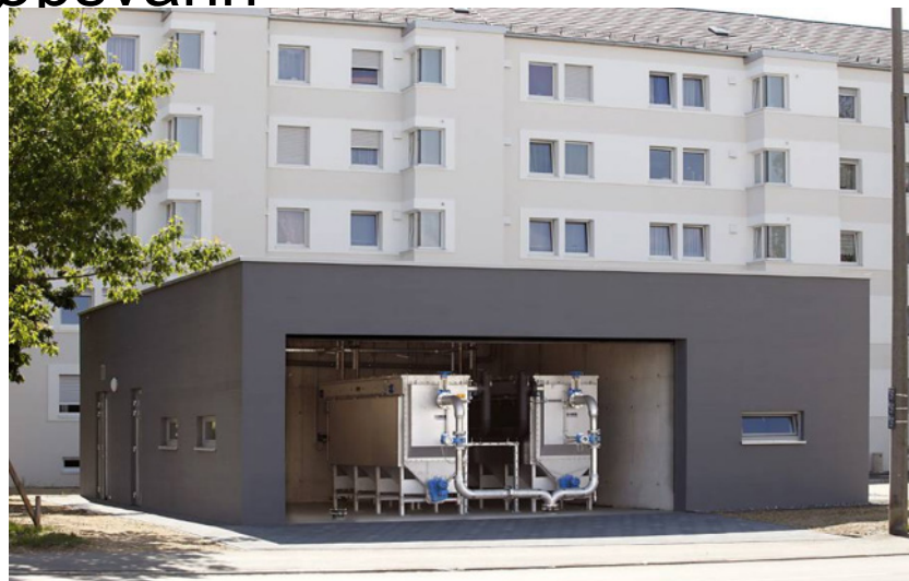
HUBER Heat Exchanger RoWin installed in a building
