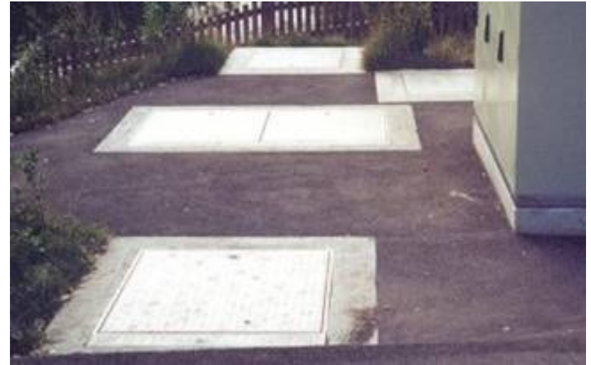
Manhole covers SD 8: back-up proof, load-bearing
