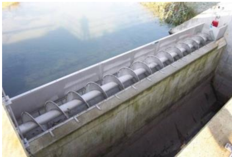
ROTAMAT® Storm Screen RoK 1 at an overflow discharge
