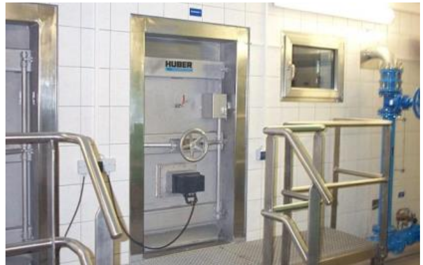
Pressure door TT 7 with central lock and spotlight
