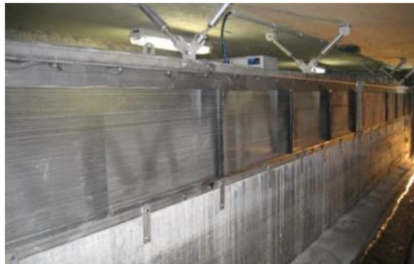
HUBER High Performance Flow Screen HSW: for treatment of 10.000 l/s storm water
