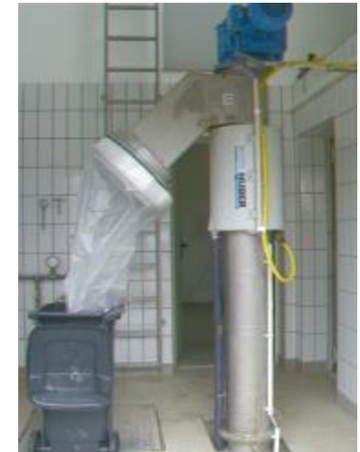
RoK 4 Screen for Baar pumping station (Germany)
