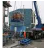
2008 Installation of subsea compressor at K-lab
