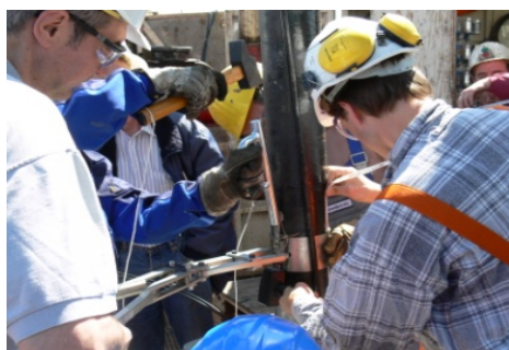
Installation of the well electrodes
