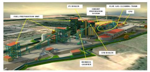
**1. CIUDEN PC boiler** is a 20MWth unit designed to applied clean coal technologies for different types of fuels (anthracite, bituminous, sub-bituminous, pet coke/anthracite mixture). The boiler allows the operation under both conventional mode (air as oxidant) and oxy combustion mode. The boiler is also designed to operate up to 25% of its thermal power provided by biomass.
