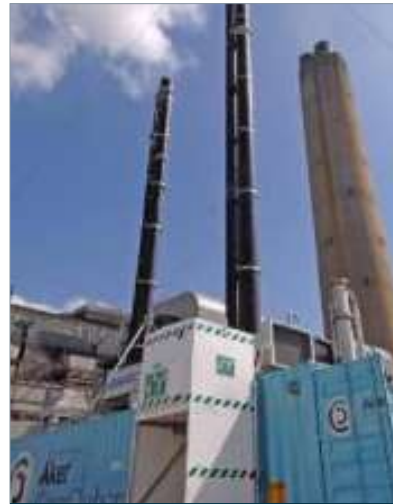
Longannet Power Plant Scotland
