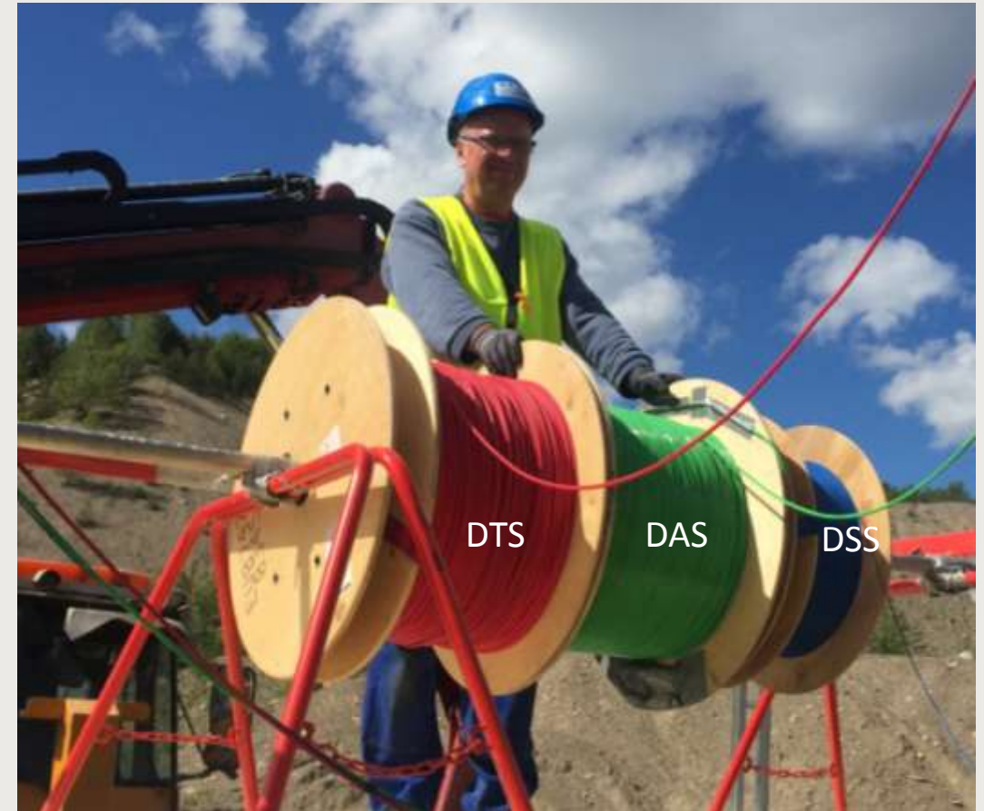
Loop installation with no splicing
