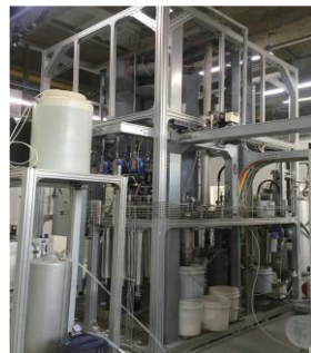
20 Nm 3 /hr scale operation with restricted heat exchange
