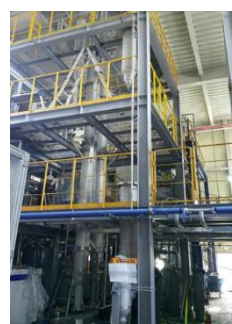
100 Nm 3 /hr scale operation with improved heat exchange
