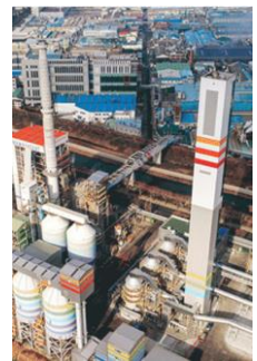
0.5MW pilot test with real flue gas (Target : 2.5 GJ/tCO 2 )
