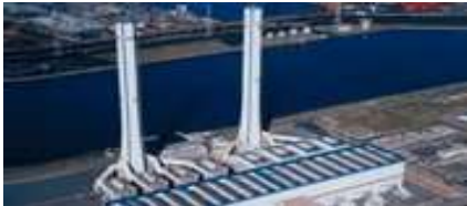
GTCC Power Plant
