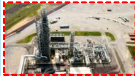
Flue gas CO 2 Recovery
