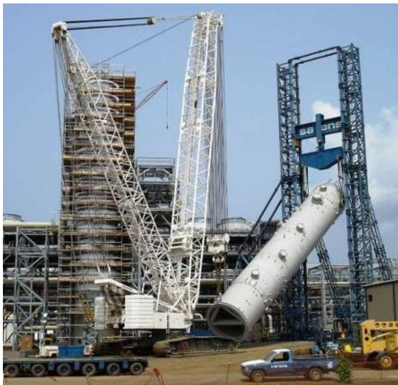
Figure 7-1: Reactor installation with gantry crane (example)
