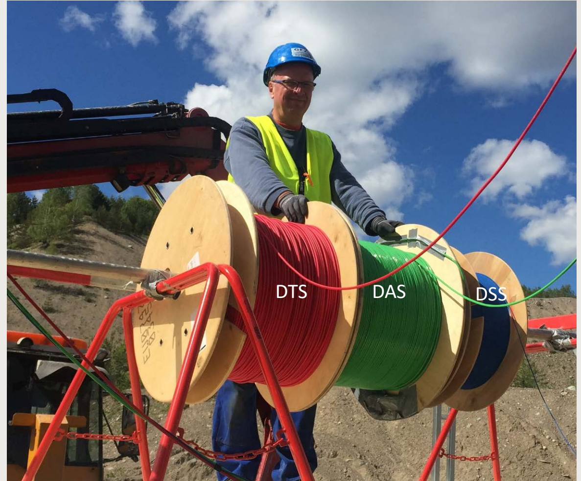
Loop installation with no splicing
