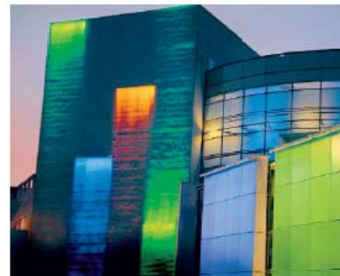
Lighting and Displays
