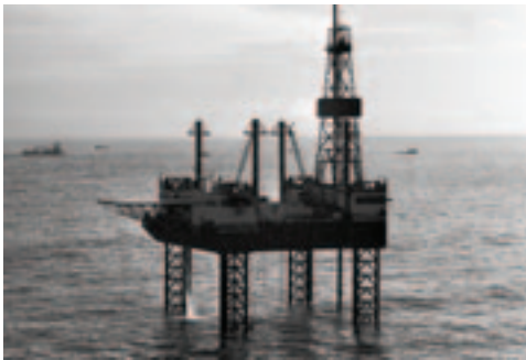
SMALL TO BEGIN WITH: Norway's first offshore installation, the temporary production platform Gulftide, commenced production in summer 1971 on Ekofisk, at depths of 70–75 metres. The rig was removed as early as 1974. Photo: Scanpix
