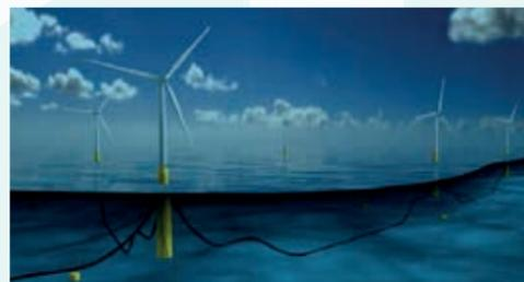
Statoil is now taking the floating wind turbine concept, Hywind, to the next step with a 30 MW pilot wind farm to be installed in Scotland in 2017. Ill: Statoil.
