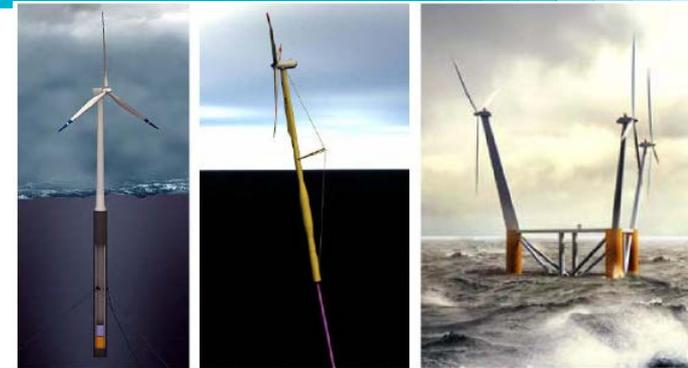
Fig. 1: Floating concepts, from left: HyWind, SWAY and WindSea.
