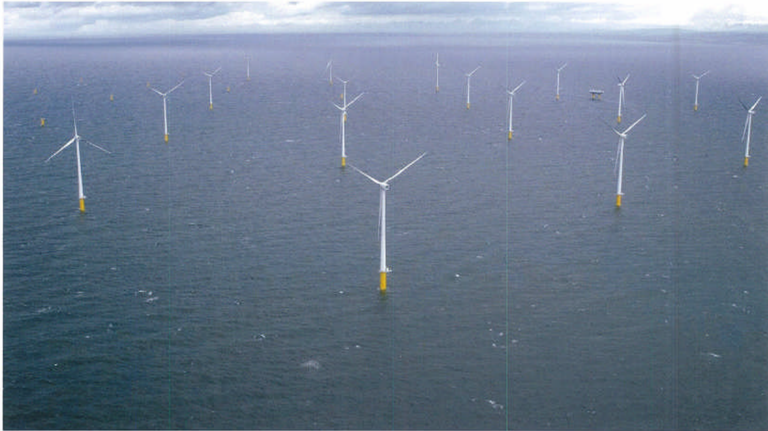
Picture taken at E.ON Offshore Project - Robin Rigg (United Kingdom, 2009)
