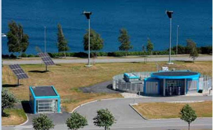
Figure 5 Energy park and hydrogen refuelling station at Statoil's Research Centre in Porsgrunn. Photograph: Ragnar Balterød, BIS Production Partner
