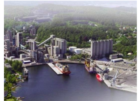
Norcem Cement Plant
