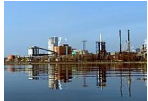
Yara Ammonia Plant
