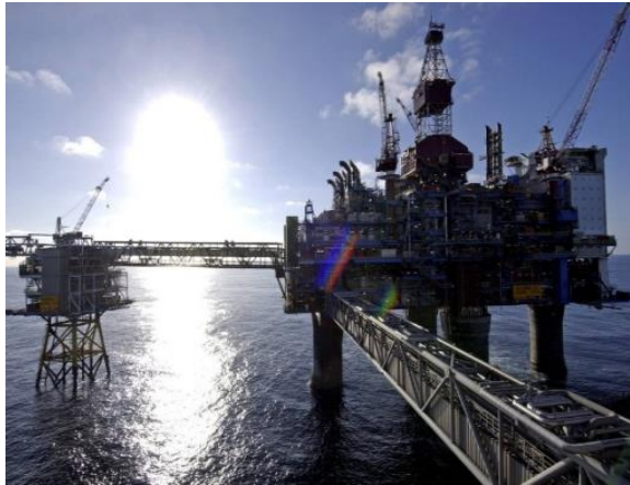
Sleipner CCS Project
