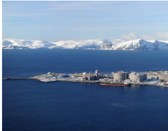
Snøhvit CCS Project
