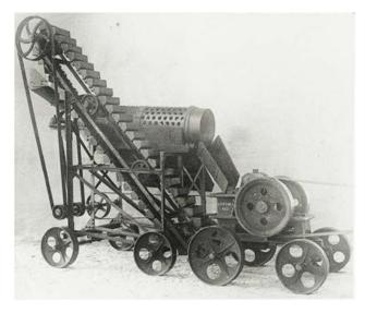
Figure 18: Mobile crushing and screening plant from the early days.
