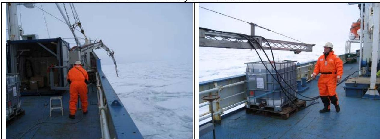
*Figure 5.2 Rigging and functionality testing/calibration of the spray arm on the R/V Lance on May 12<sup>th</sup>.*
