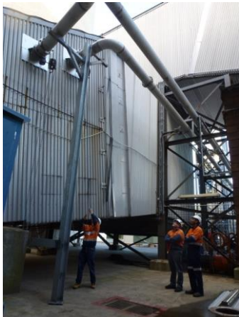
Opening of real flue gas to test unit for first time at Vales Point Power Station
