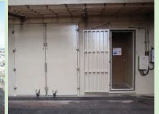
Watertight door that prevents water intrusion into the building
