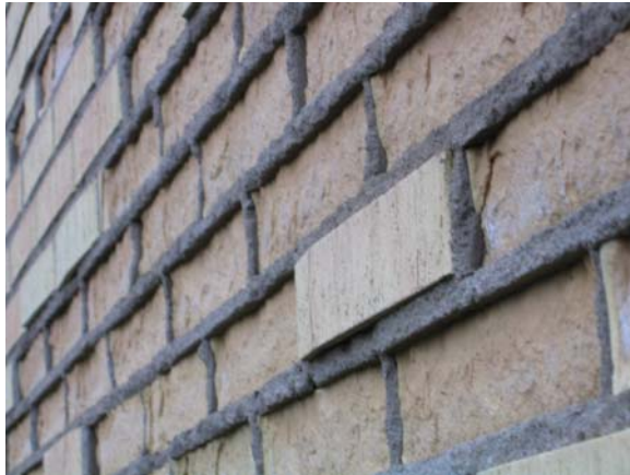
Figure 3 Brick façade before renovation
