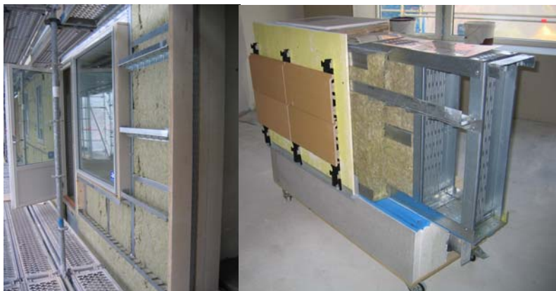
Figure 4 Outer long side wall construction
