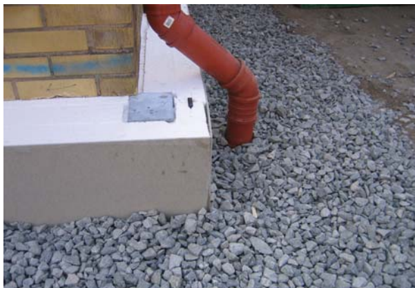
Figure 2 Outer eps insulation on slab on the ground
