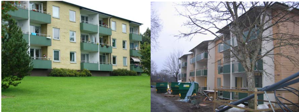
Figure 6 Balcony construction before and after renovation
