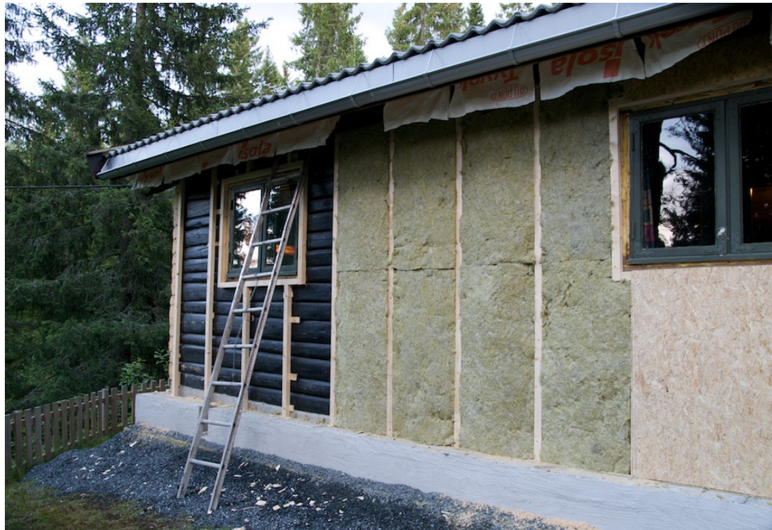
Installation of the insulating facade
