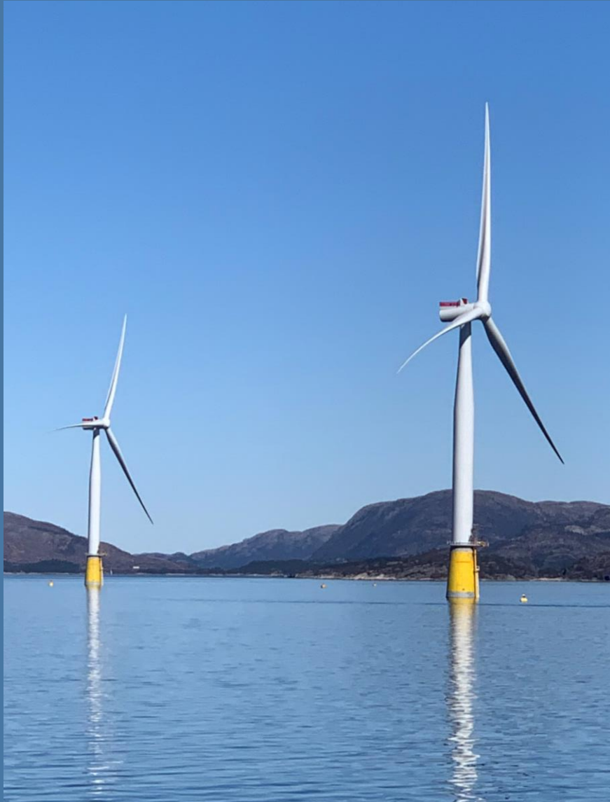
Turbines in Hywind Tampen, Norway [own photography]
