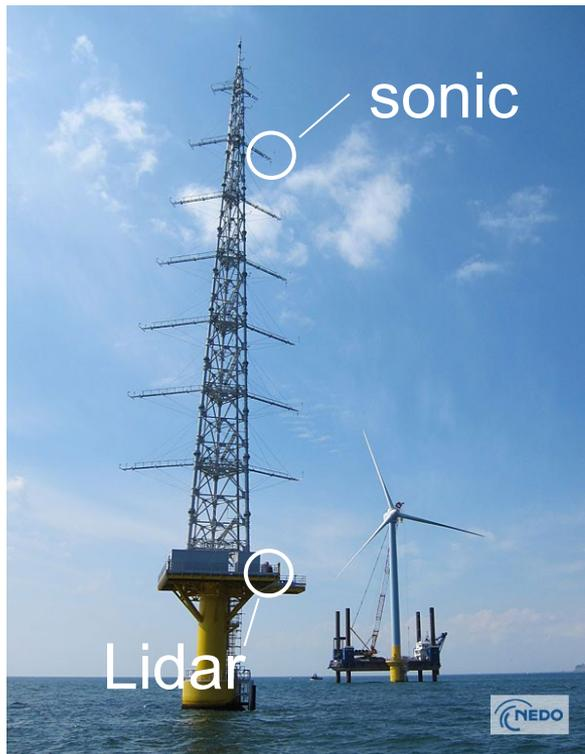
Measurement data at Choshi offshore met mast was used for validation
