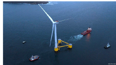
Figure 1 Tow-out of WindFloat Atlantic FWT. Source: EDP Renewables [1].
