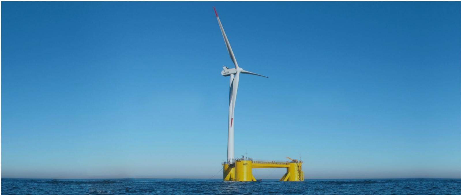
The Windfloat pioneer FOWT, from Principle Power Inc, deployed in Portugal.
