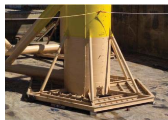
Close-up of a heave plate used on Principle Power's WindFloat platform; and platform assembly near Lisbon, Portugal; (Antonutti, et al. 2014)
