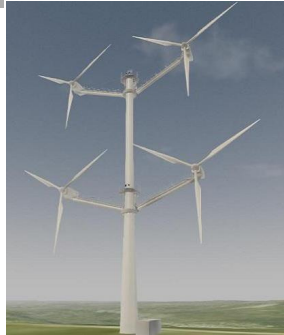
Vestas 4-rotor demonstrator turbine. Source: Vestas ( www.vestas.com )
